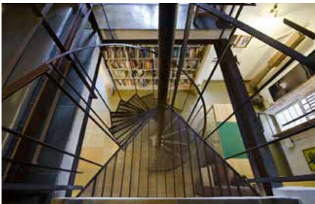
Figure 8: Spiral Staircase leading to the loft (Source: https://localground.in/work/studio-877/ )
