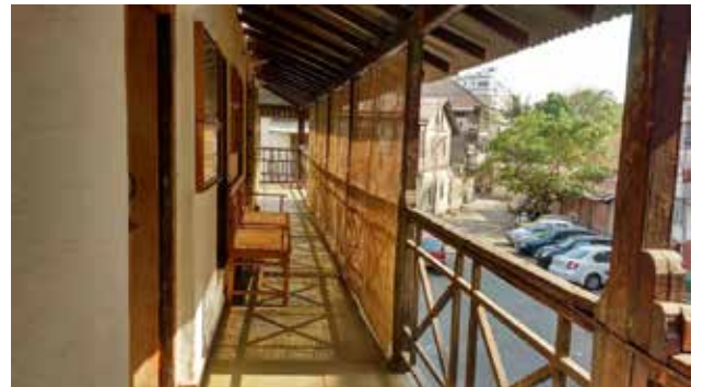
Figure 5: Corridor (Source: https://localground.in/work/studio-877/ )
