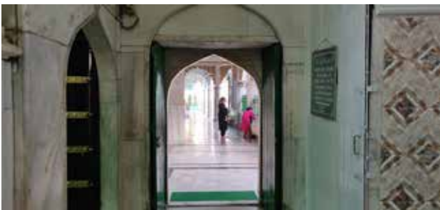
Figure 9: Tiling done on the Dargah by the committee- an insensitive intervention. (Source: Author)
