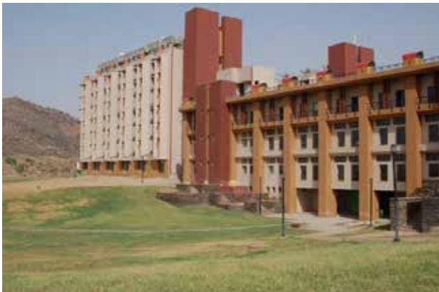
Figure 8: N.I.I.T Neemrana Campus with PDEC and peripheral exhaust shafts (Source: Gupta, 2014)
